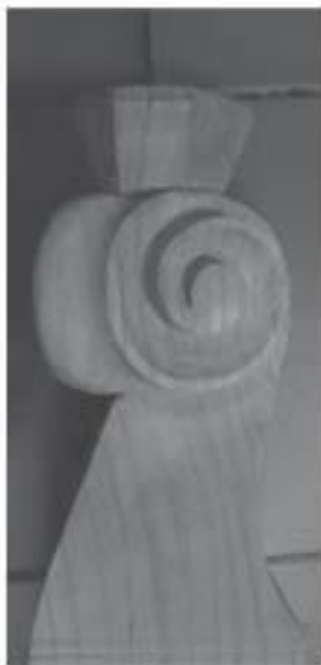
Closer view of the molding
